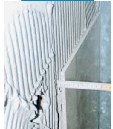
Thickly applied porcelain tiles on a wall
