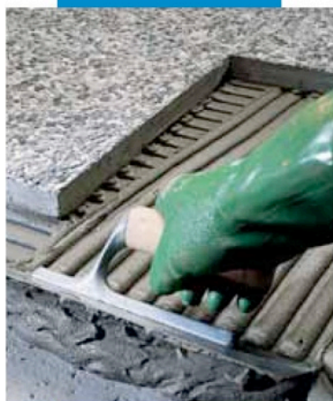
External installation of relief terrazzo "graniglie" tiles
